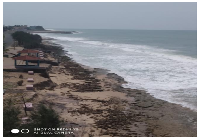
Fig-1 Structural Erosion in Sangudurai Beach
