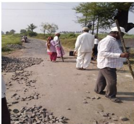
Figure 4 Road Construct Sapkalwadi village
