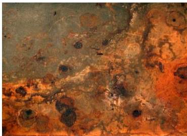
Fig-5 Pitting Corrosion Behaviour of steel
