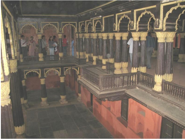
Fig. 3. Balcony and Corridor (Before)
