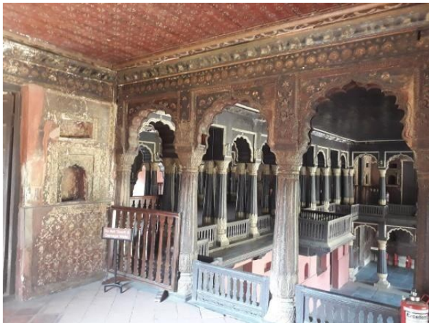
Fig. 4. Balcony and Verandah (After)
