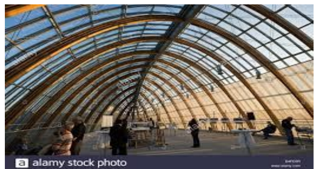
Fig. 7- Barrel vault rooflight
