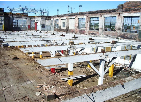
Fig 4-Deconstruction of a commercial building
