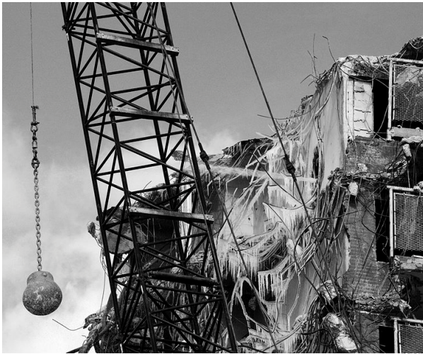
Fig 2-A wrecking ball in action at the demolition of the Rockwell Gardens
