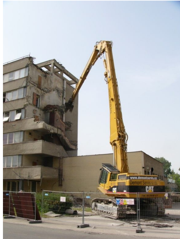
Fig 1-A high reach excavator during demolition
