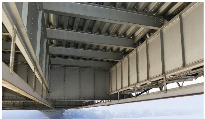
Fig. 22: Underside of the Bridge Deck
