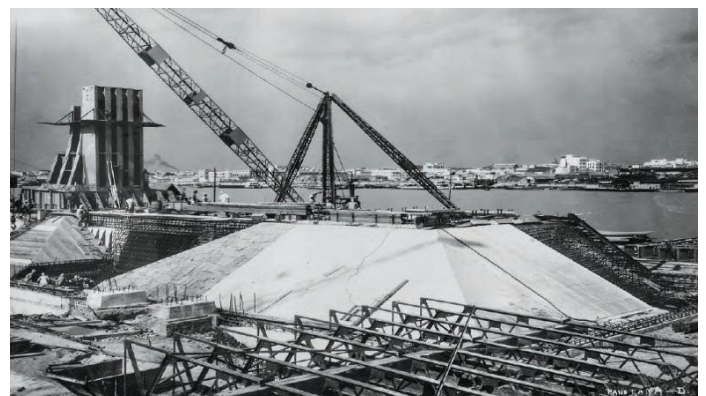
Fig. 5: Constructions of Superstructure in progress
