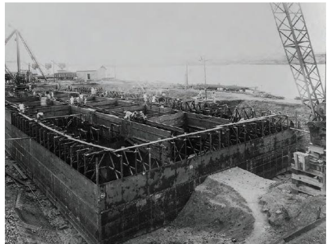
Fig. 4: Constructions of Abutments in progress
