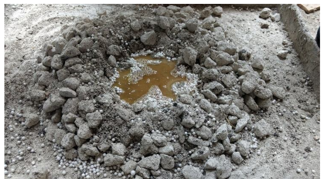
Fig. 5 mixing of all the ingredients of light weight geopolymer concrete
