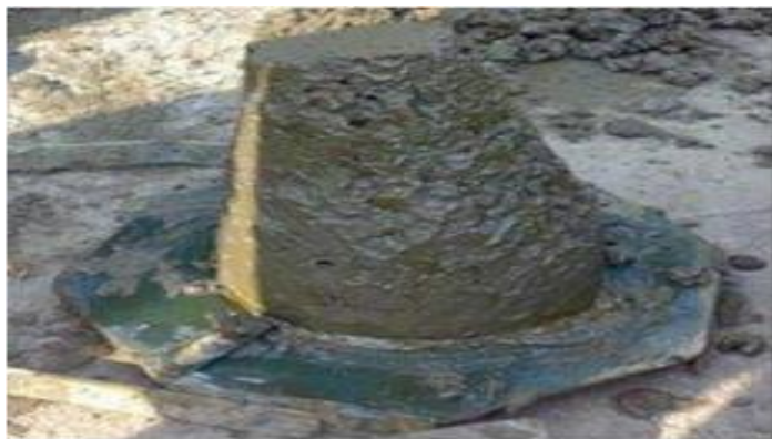
Slump cone test
