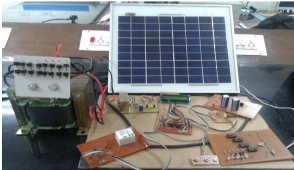
Fig.6 Hardware Model of Charging Station
