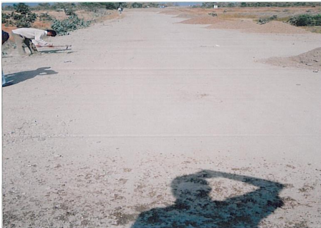
Fig. 5.1 Preparation of subgrade for laying of Jute Geotextile
