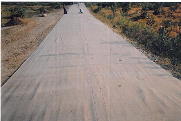
Fig. 5.2 Laying of Jute Geotextile on one side of the prepared subgrade
