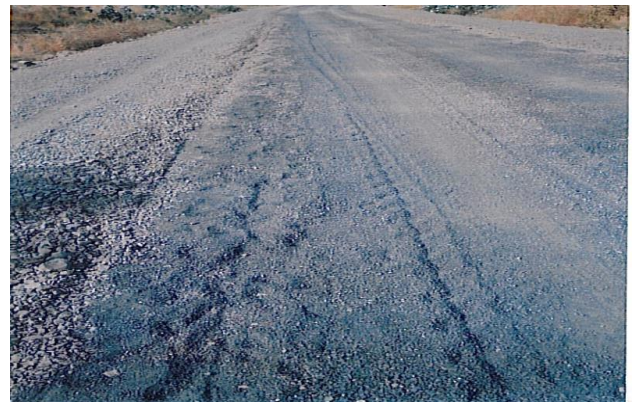
Fig. 5.5 Rolled surface of subbase over Jute Geotextile
