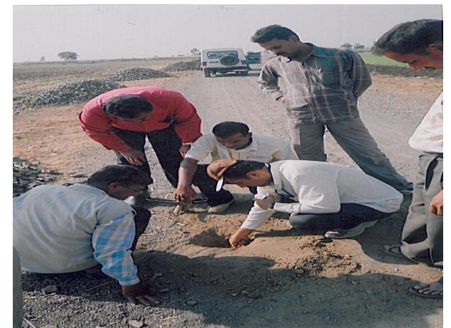
Fig. 5.6 Checking the condition and position of Jute Geotextile by taking sample
