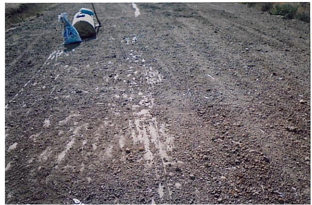
Fig. 5.4 Laying of sand cushion on the Jute Geotextile
