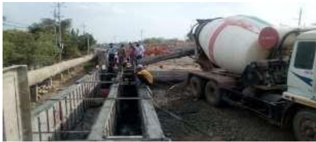
Fig -1: Discharging of RMC at project Site
