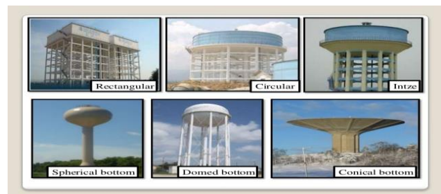
Fig 1 Types of overhead water tank
