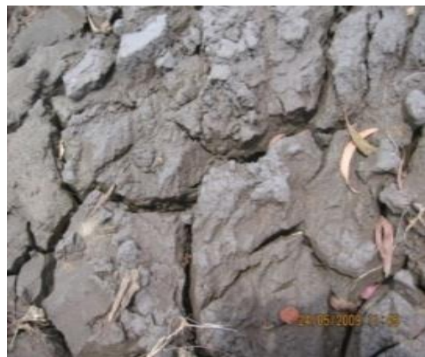
Figure1 Marine Clay Showing Cracks
