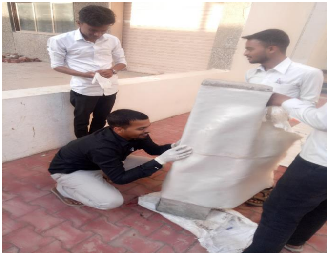
Figure.6 – Retrofitting of RC Beam by GFRP Sheets
