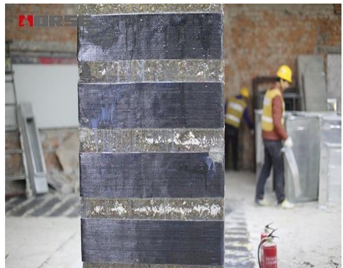
Figure.5 – Wrapping of CFRP Sheets on Column
