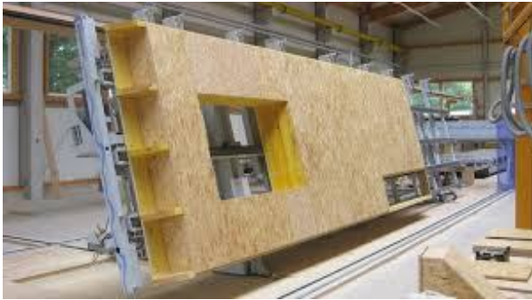
Fig 2 prefabrication In Housing Construction
