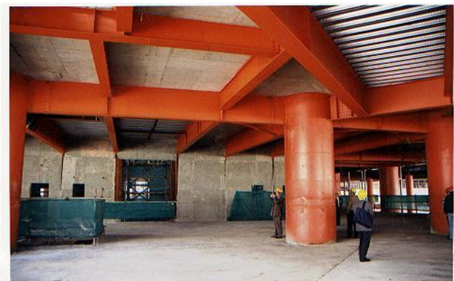
Fig. no1.4 Composite steel story system
