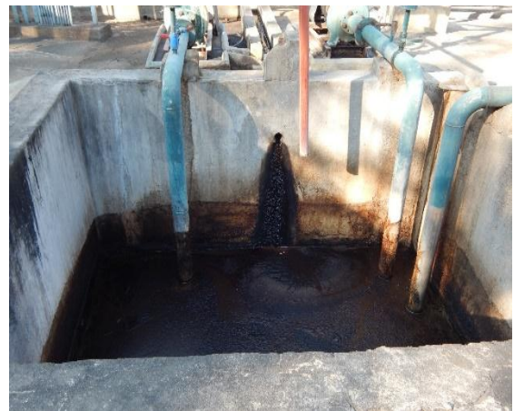
Fig 1: Image Showing Hot Spent Wash Storage Tank
