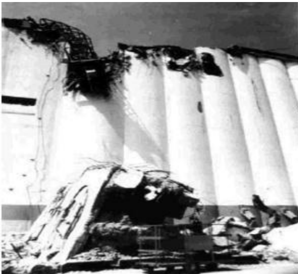
Fig. 1 Partial collapse of grain silo during 1974 Lima, Peru earthquake
