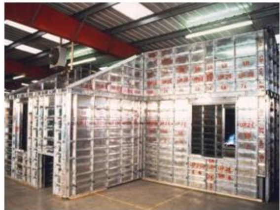
Fig 2.1 .Mivan formwork
