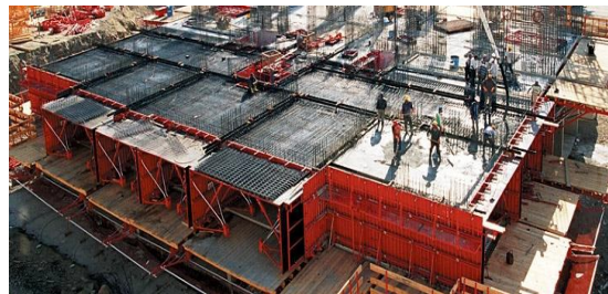
Fig 2.3 Aluminium Formwork during construction
