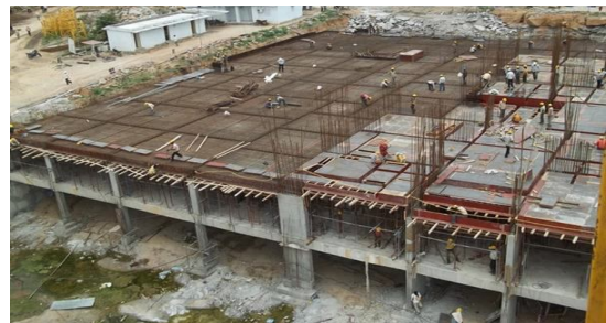
Fig 2.2 Aluminium Formwork during construction
