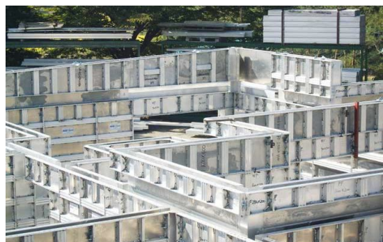
Fig 2.4 Aluminium Formwork during construction
