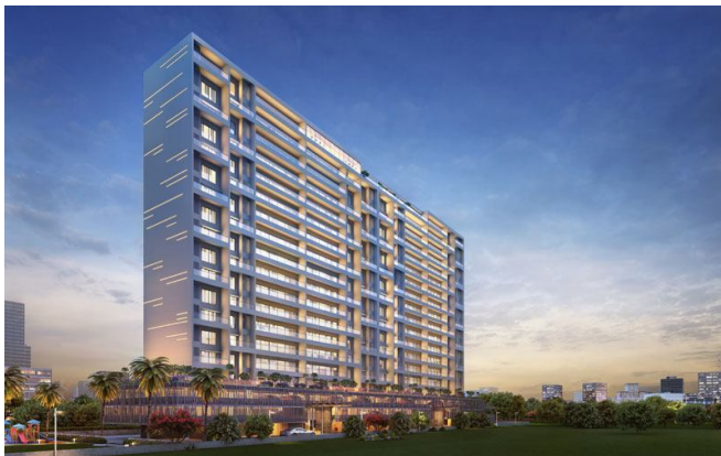
Fig 1: 3rd eye view of actual site
