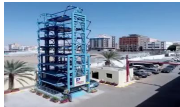
Fig3.12 : 3rdEye View Of Actual Site
