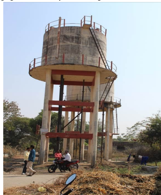
Fig. 3 Elevated Storage Reservoir
