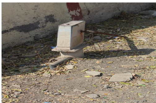
Fig. 10 Damaged Handpump
