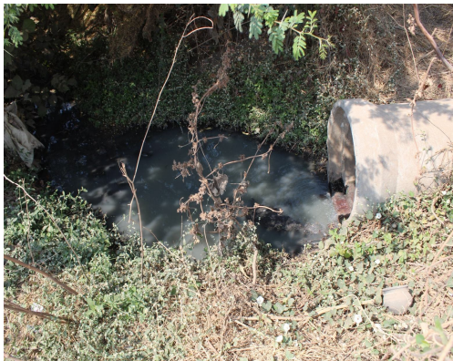
Fig. 9 Outlet of sewer
