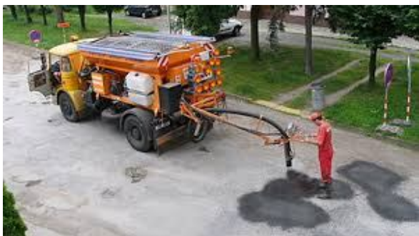
Figure 6- Pothole repairs
