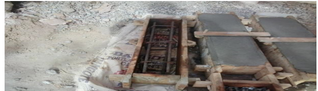
Figure 3: concrete in mould
