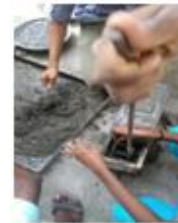
Figure 13: Compacting
