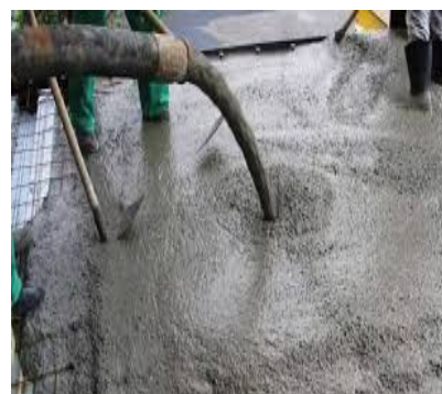
SELF- COMPACTED CONCRETE
