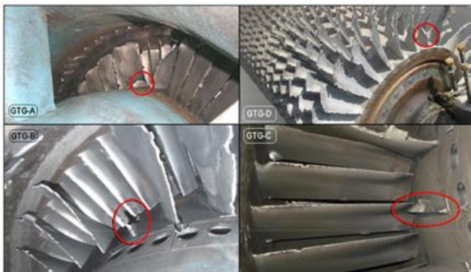
Fig. 1 Failed blades in first row of four frame-6 gas turbines
