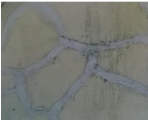
Treated Surface with Crack-X Paste
