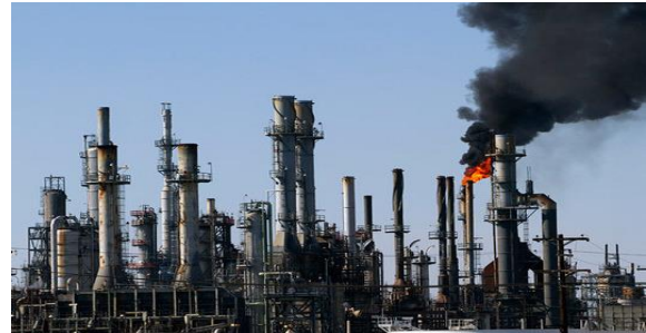
Figure 1.1 Industrial Steel Chimneys (Ref: www.vedomosti.ru )
