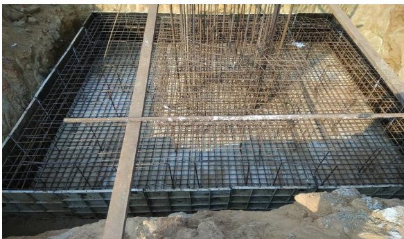
Fig-8 Placing of reinforcement bars
