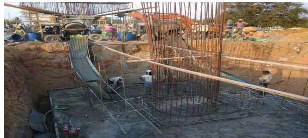
Fig-10 (a) : Placing of concrete
