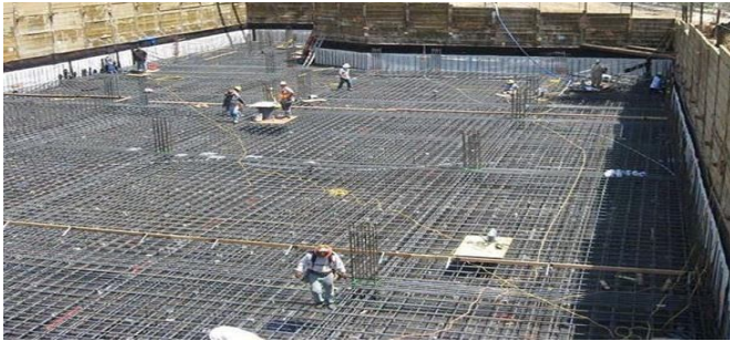
Fig-5: Raft Foundation
