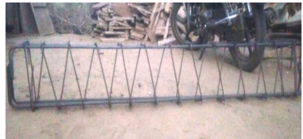
Fig.1 Rectangular Spiral Reinforcement.
