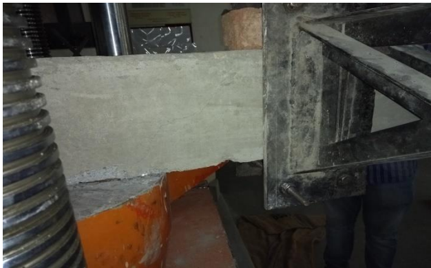
Fig.5 Crack pattern of control beam
