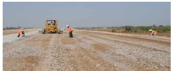
Fig 17 Laying of granular sub base layer (GSB)
