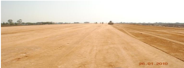
Fig 18 Subgrade preparation
