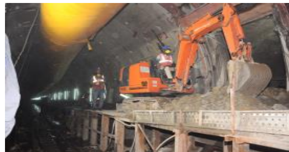
Photo 2: Mini Excavator working over Platform
