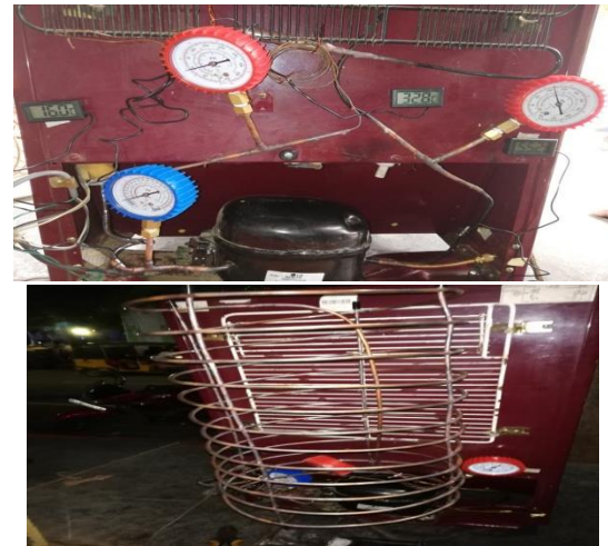
Figure 7. existing condenser and modeled condenser
