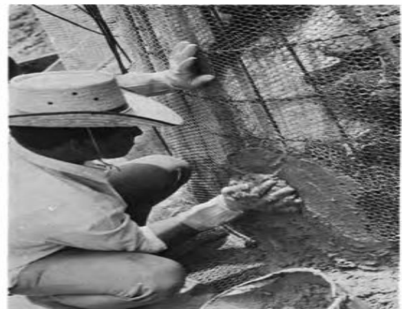
Fig1.4: A paste of mortar is forced into the layers of mesh by hand . . . (Smith Kam· pempool, Applied Scientific Research Corporation of Thailand)
