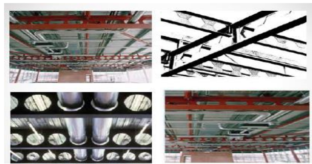
Figure.1 Application of beams with web openings
