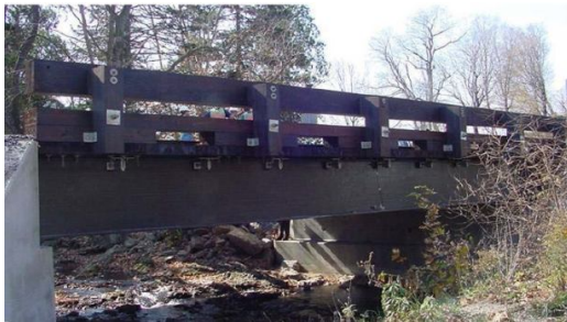
Figure 2. Double Web Beam With Stiffeners
