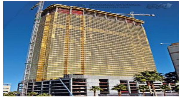
Figure 1.2: Flat Slab Post-Tensioning of High-Rise Building in Las Vegas
