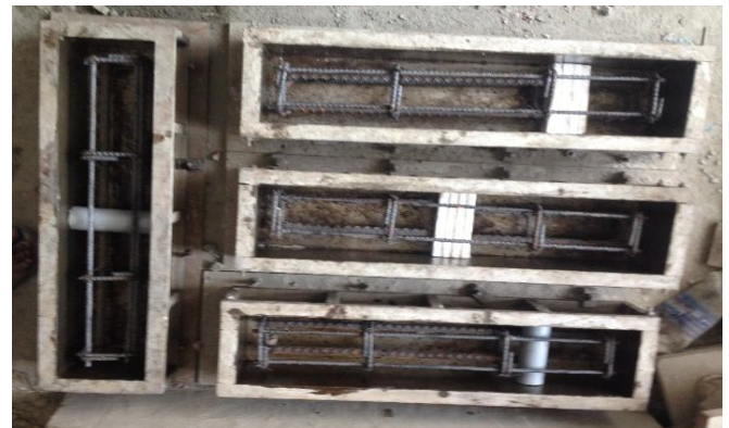
Figure 1: Placing of Openings and Cutouts.
