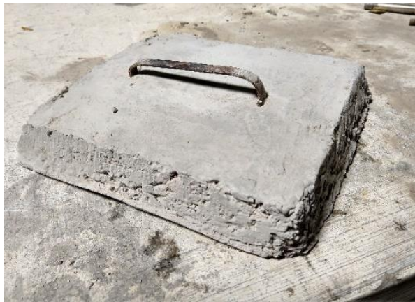
Fig 9: Inspection chamber cover
