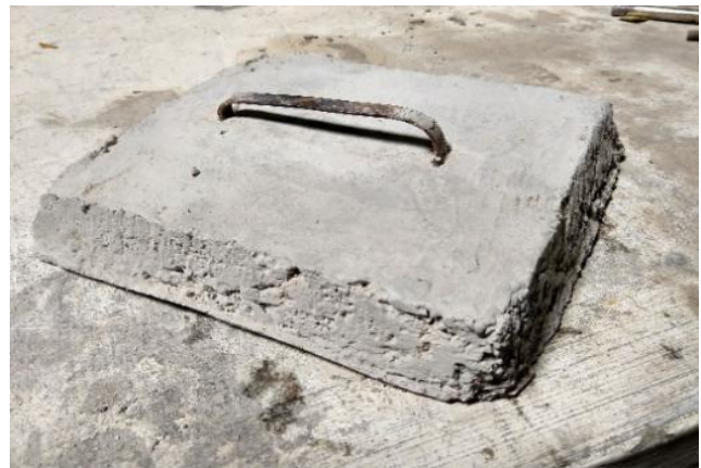
Fig 9: Inspection chamber cover
