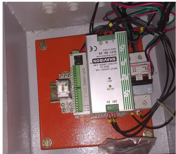
Fig : 4 PLC connection with relay
