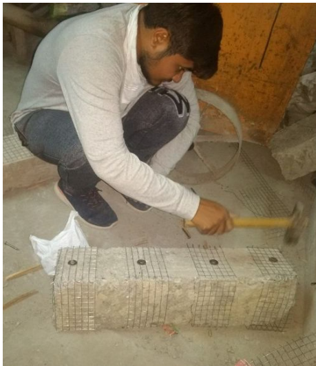
Fig 8 Strip wrapping using wiremesh
