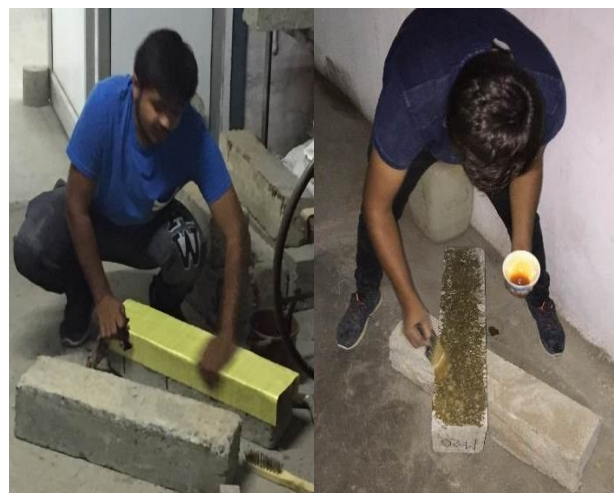
Fig 5 Appling resin and AFRP sheet
