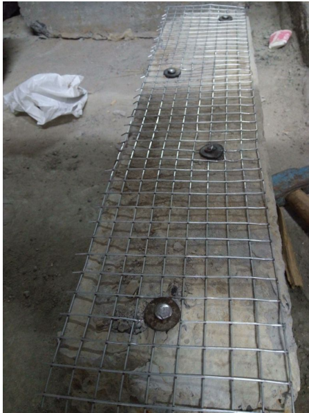
Fig 7 Retrofitting of beam using wiremesh.
