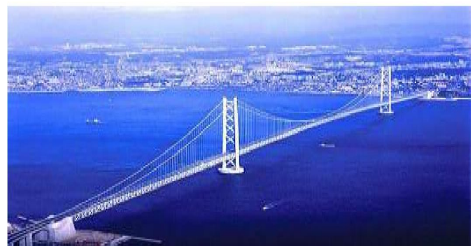
Fig -1: Akashi Kaikyo Bridge (Japan)
