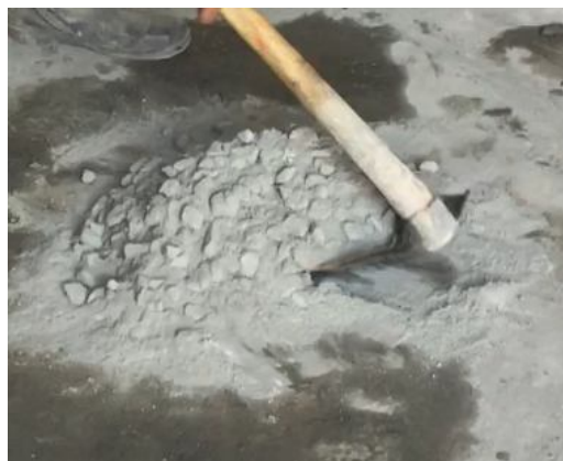
Figure. 3 mixing of concret
