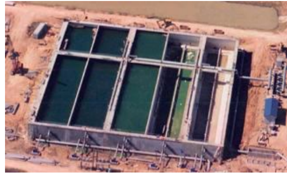
Fig 1.1.9 Rectangular Water Tank
