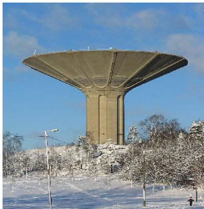
Fig 1.1.8 Conical Water Tank
