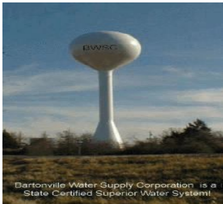
Fig 1.1.11 Spherical Water Tank
