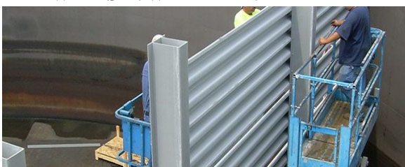
Fig.1.1.13 Baffle Walls in Water Tank
