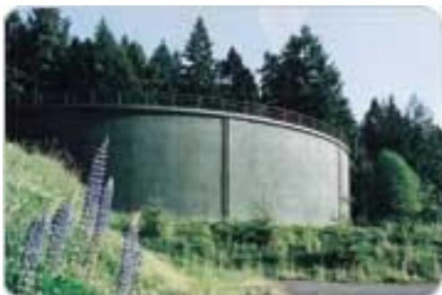
Fig 1.1.3 Tank Resting on Ground
