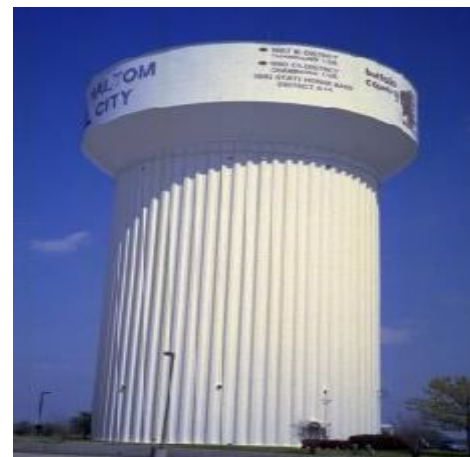
Fig 1.1.6 Overhead Water Tank
