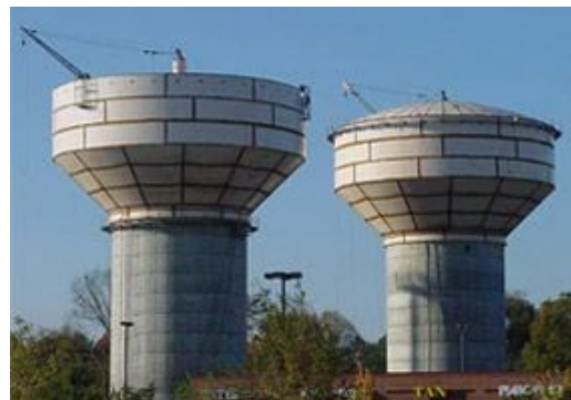
Fig 1.1.10 Intze Water Tank
