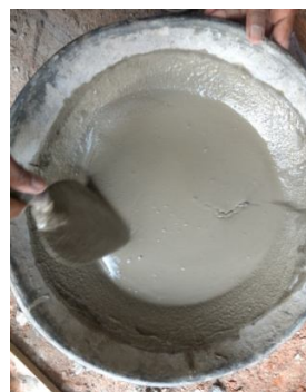
Fig 3: mixing of cement slurry
