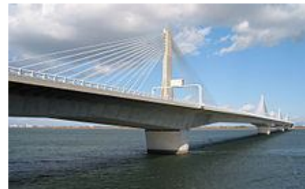
The Twinkle-Kisogawa is an extradosed design, with long gaps between the cable supported sections.
