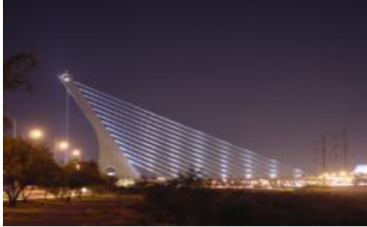
Puente de la Unidad, joining San Pedro Garza García and Monterrey, a Cantilever spar cable-stayed bridge
