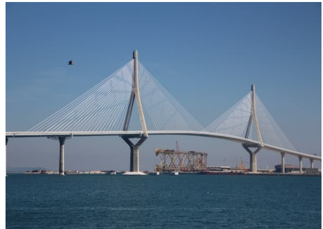
Figure no.1: suspension cable stayed bridge
