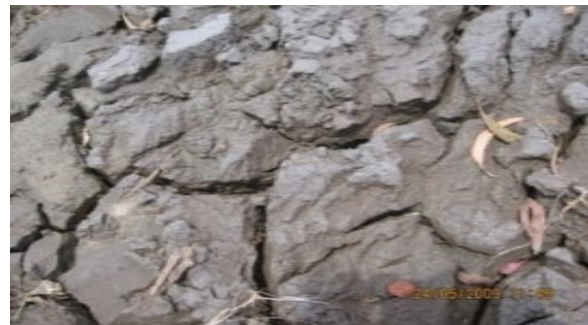
Fig 2.2 Cracks in Marine Clay Deposits
